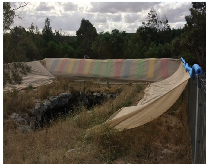
Figure 4. Additional padding on the smooth metal panel in the form of (colourful) inflated air mattresses and pool noodles on the top of fence. Photo: Yvonne Ingeme
