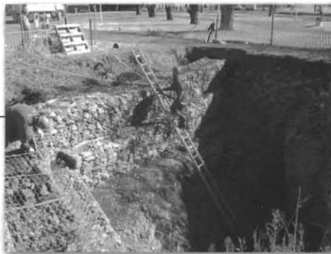
All Gabions now filled and in place.
