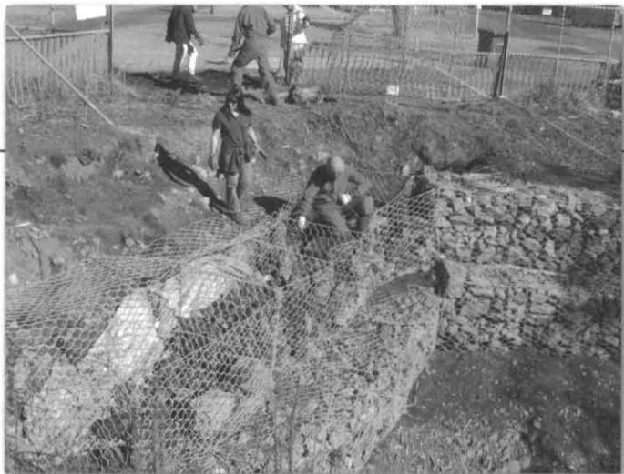
Top row of wire Gabions in position.
