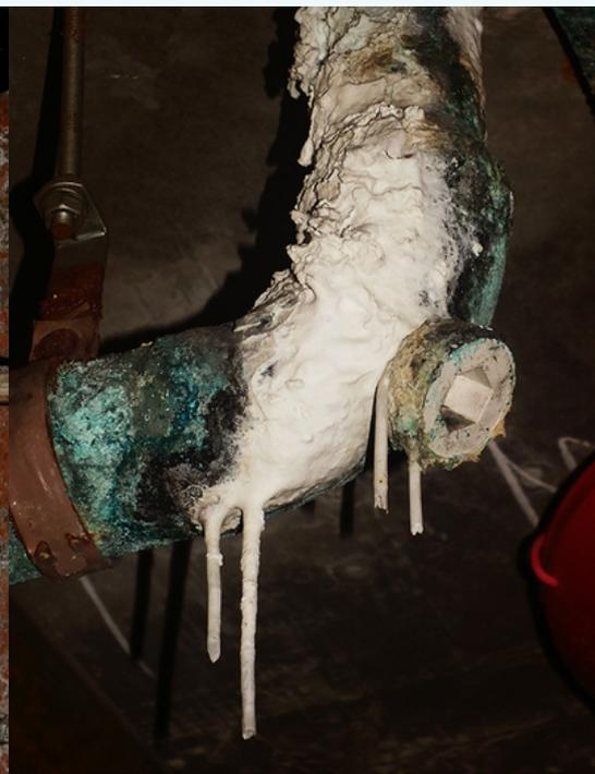
Fig 6. Calthemite flowstone and straws on pipework
