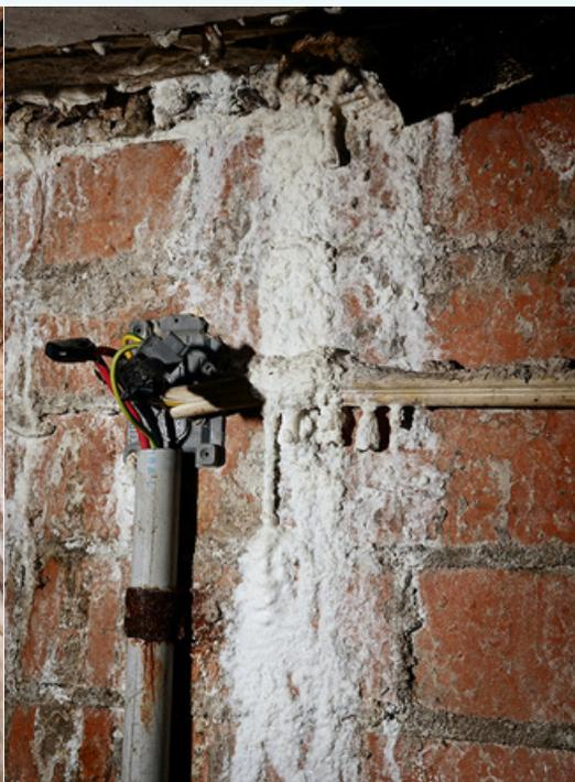
Fig 5. Calthemite deposits on electrical wiring under building
