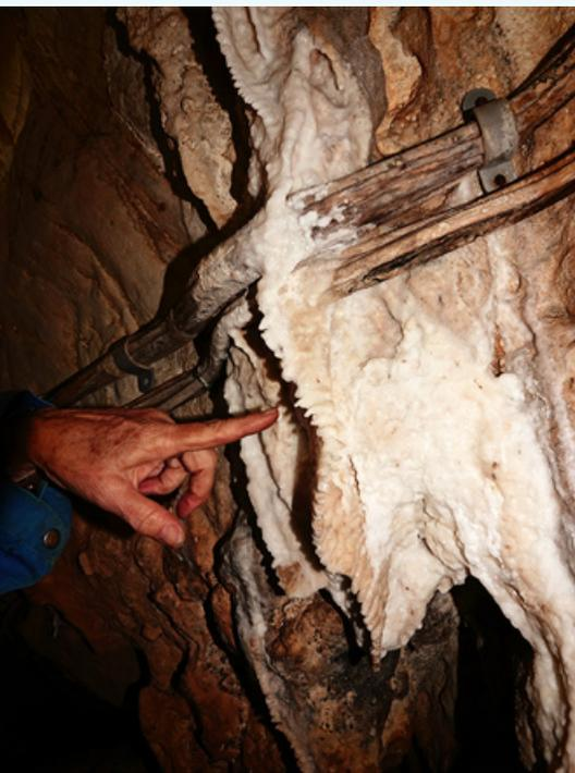
Fig 4. Calcite over the power cables in Hill Cave, Abercrombie, NSW
