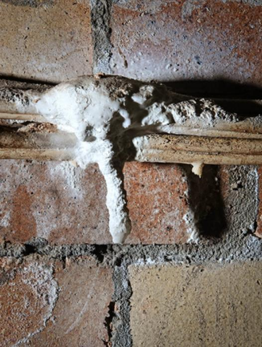
Fig 7. Calthemite stalactite attached to electrical wiring
