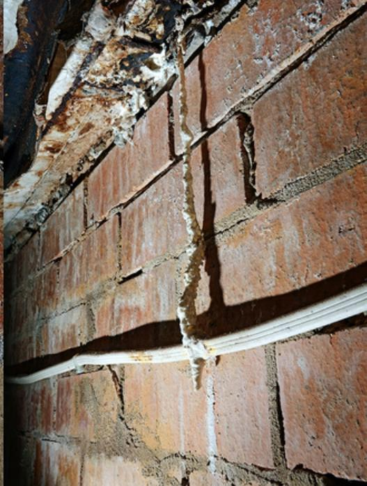
Fig 8. Calthemite column & stalactite on electrical wiring
