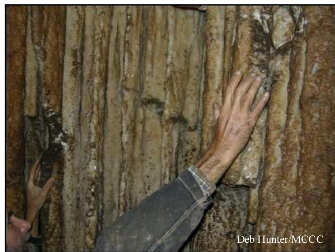
*Helictite Cave: More damage, Tom Porritt (CCC) shows foot holds cut into the crystal wall.*
