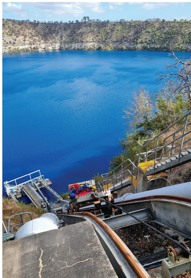
The gantry and pontoon showing the remotely-operated gear trolley, which assisted in delivering gear to the lake surface. Picture: Mark Simpson
