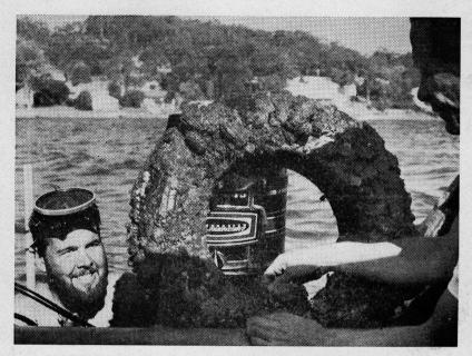
• "This is what an old car tyre looks like after two years on the bottom," John Matthews tells Dr. Bruce Malcolm, both of the New South Wales Fisheries. This is one of the tyres put on the bottom as a preliminary to the laying of the artificial reef. When covered with marine growth, like this one, the tyres will attract more fish to Lake Macquarie, N.S.W., and improve fishermen's catches
