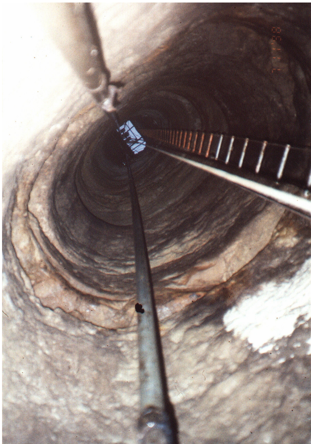
Looking up the shaft of 5L412c
