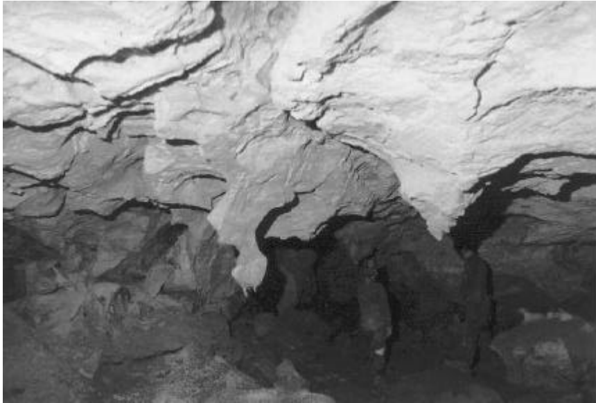
The start of the Railway Tunnel.
