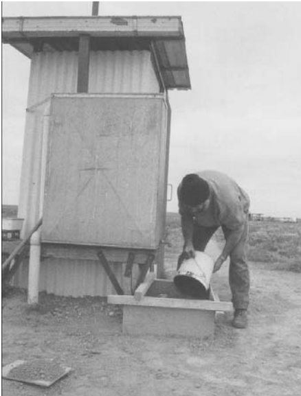
Ray Gibbons constructing ablutions area for Old Homestead Cave toilet. Photo: Peter Ackroyd, 6 Oct 2002
