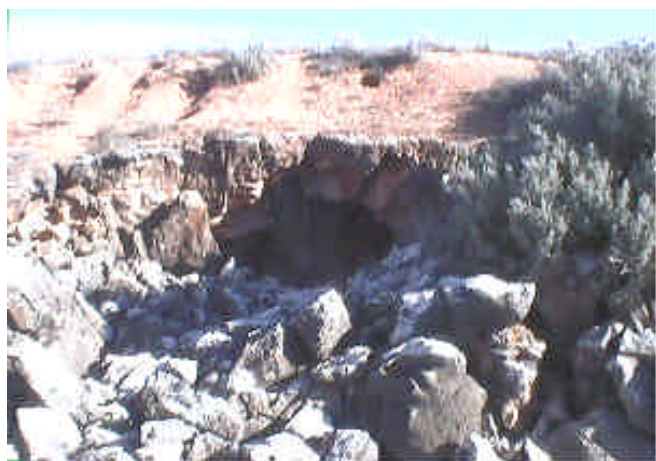
Fig. 4 N2238 Collapse Doline & Cave entrance @200deg
