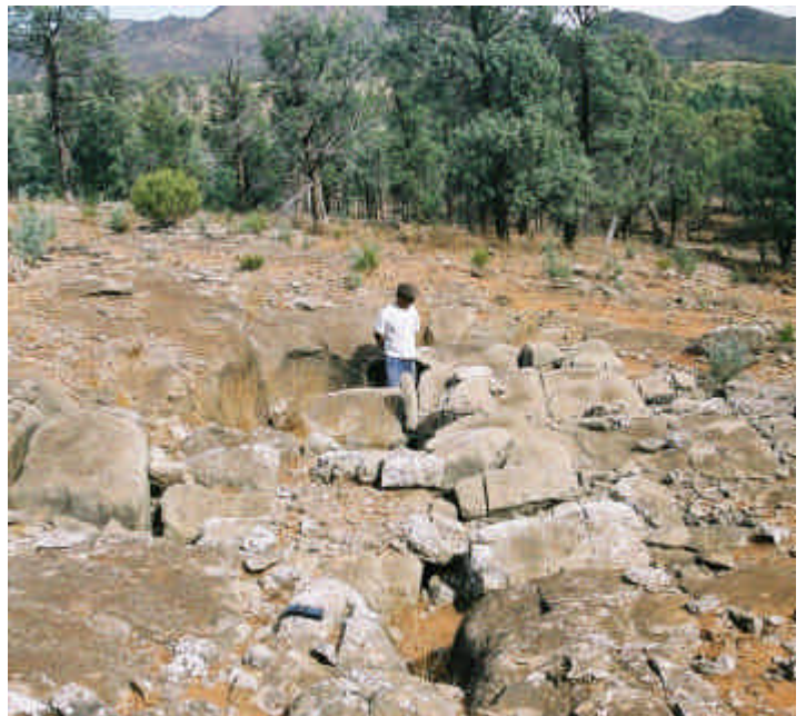
Eddie at F217 collapse (B Binks)
