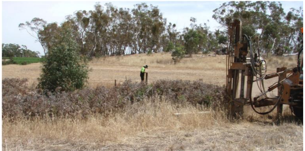
Tortoise Cave fencepost installation
