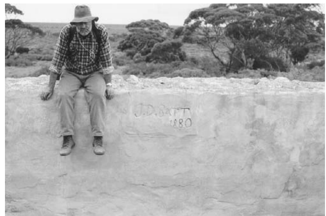
Ray Gibbons on mortar-lined rock and stone tank near Kuthala Pass. Note builder's name and date marked in the mortar, "J D Batt, 1880".
