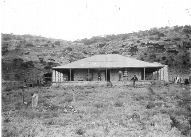
Original Madura Homestead. Photo: William Russell Evans, ca 1905. Image courtesy of the State Library of South Australia, Call No SLA: B54060/73
