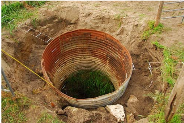
Outer tank removed and gaps around the inner tank partially back-filled.
