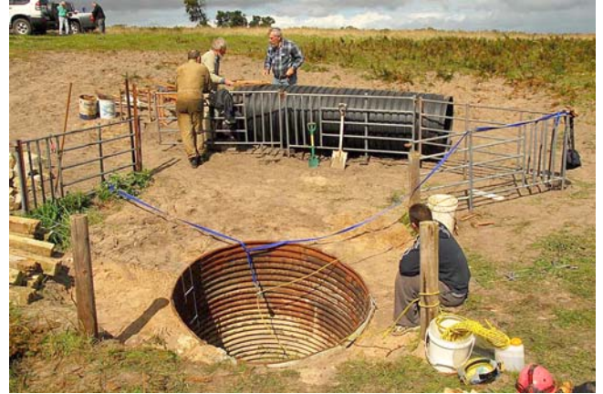
The surrounds of the inner tank are now completely back-filled. The stormwater pipe is in the background.
