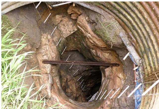
The rock around the top of the solution pipe has been cleaned. Photo: Clare Buswell.
