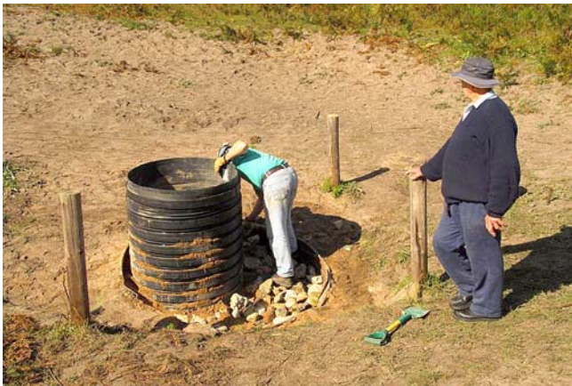
The stormwater pipe has been placed on top of the solution pipe, the surrounds at the base have been sealed with concrete and the inner tank then back-filled.
