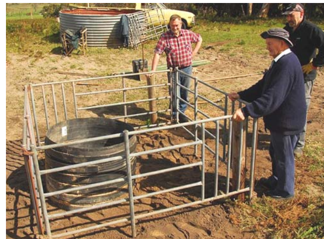
The area around the pipe has been built up with sand to the level of the surrounds. A temporary fence has been put back in place until the entrance to the pipe can be properly secured.
