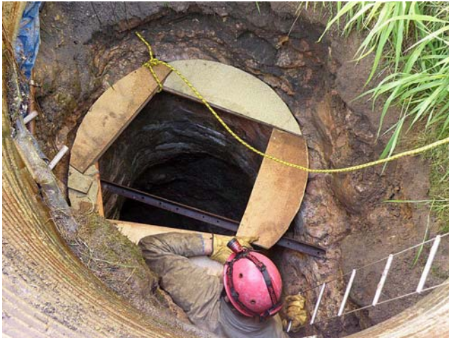
Fitting the wooden frame. Photo: Clare Buswell.
