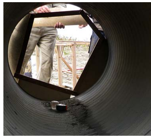
Measuring the wooden frame to fit the stormwater pipe. Photo: Clare Buswell.
