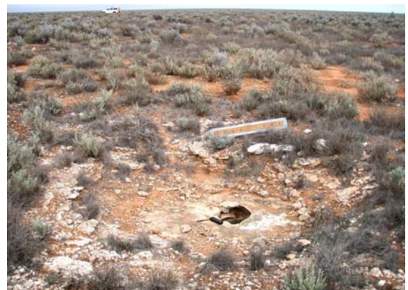
N-4388 blowhole @230 from 5m
