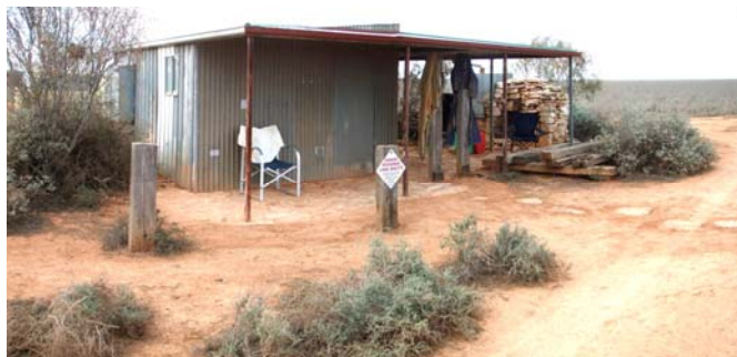
Old Homestead Hut after paving upgrade
