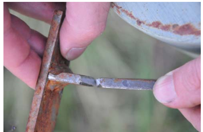
Vandalised gate locking bracket.
