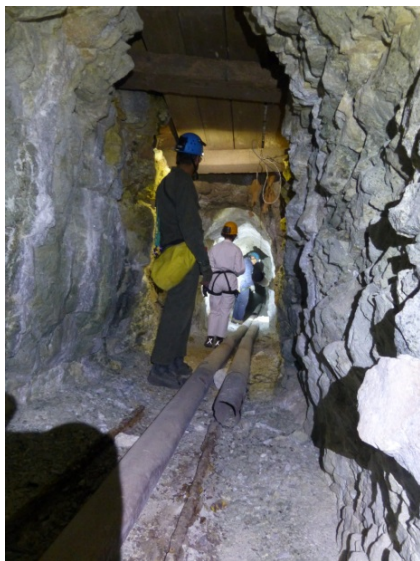
Air pipe laying silent
