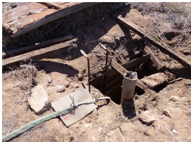
Dolomite mine entrance, showing air pipe
