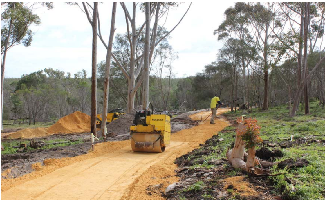
Motorised wheel-barrow on the new pathway to the Bat Observation Centre, no cave is recorded under here but the path is adjacent Peppertree doline.
