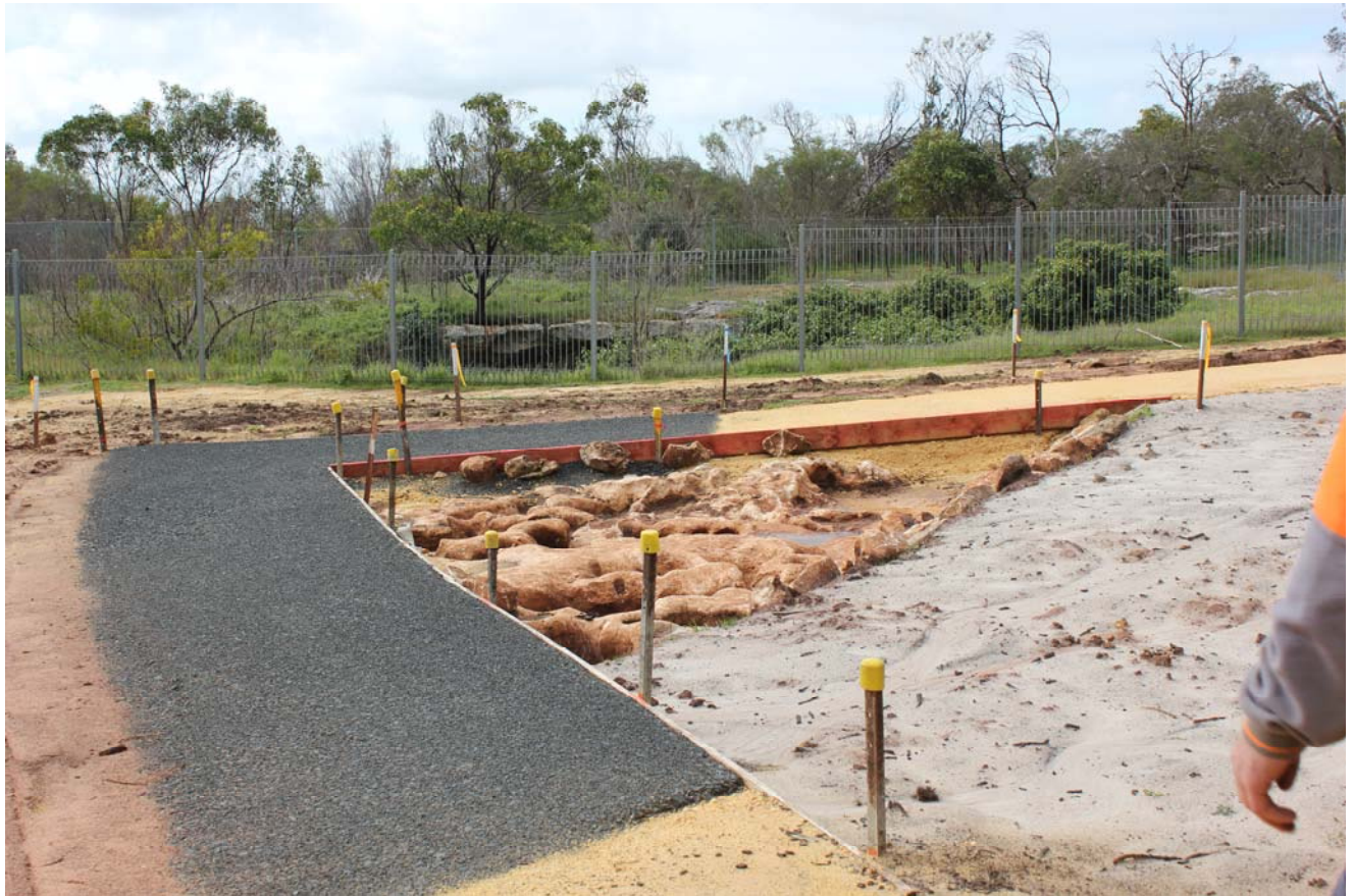
Exposed section of epikarst / pathway upgrade, adjacent Blanche Cave's third roof hole
