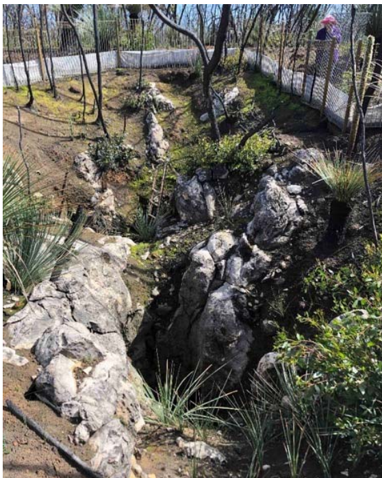
Erosion control around K1. Photo: Clare Buswell
