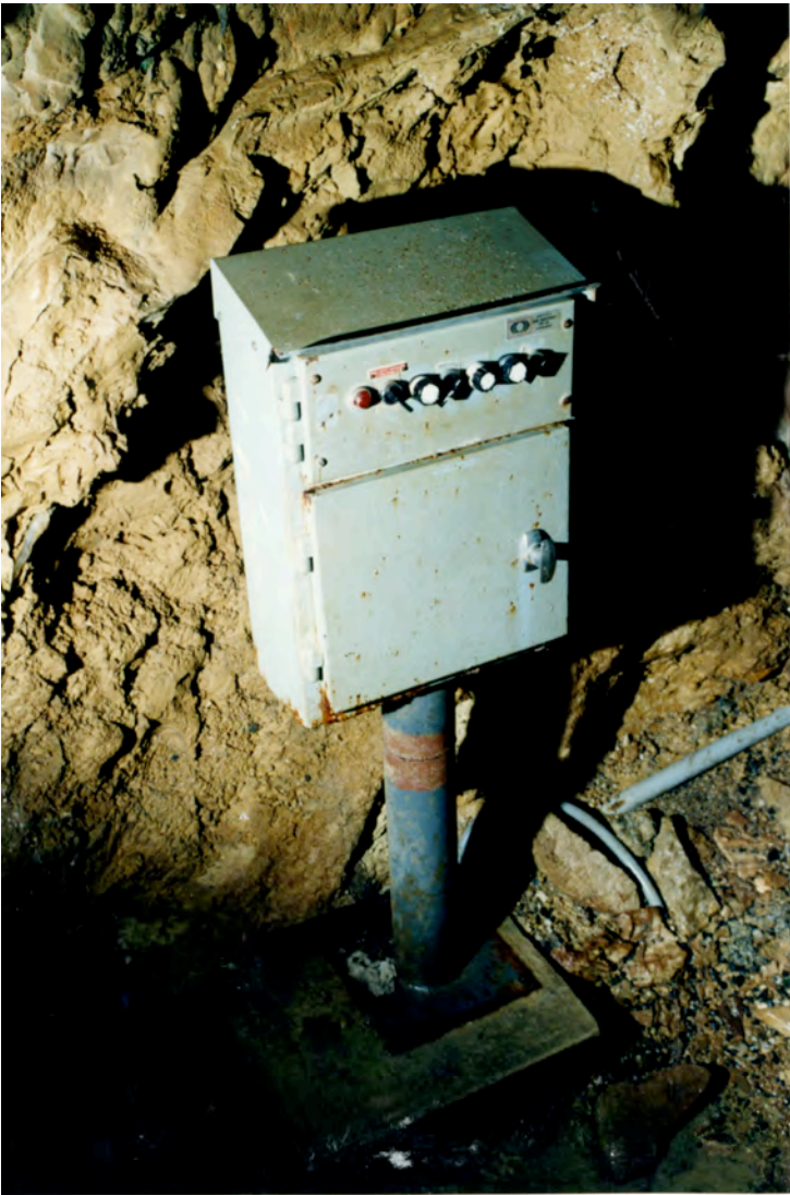
Section 2.11 Many outmoded, aesthetically obtrusive light fittings and switch stations are located throughout the cave. Environmental degradation through drilling, cable and conduit location and lampenflora growth is ongoing.
