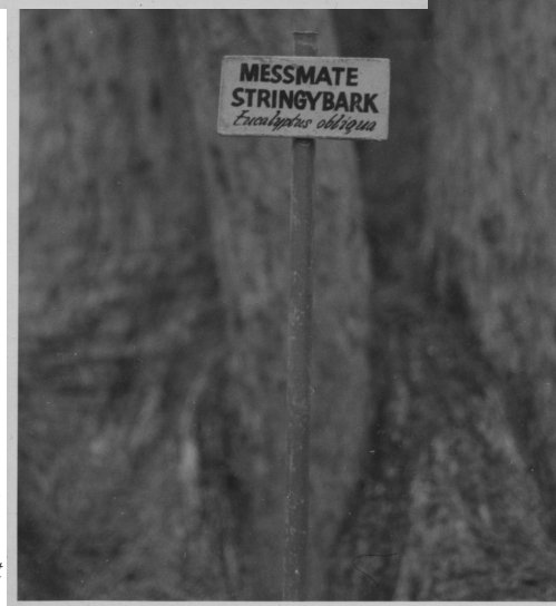
Poto 14.> Interpretive aid in Mt Field National Park. Constructed from 2 cm pipe welded onto steel plate with painted lettering.
