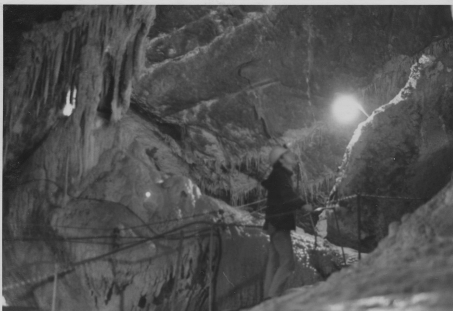
Photo 51. Overhead wiring in Marakooa Cave. Mains wiring should ideally be concealed in conduit and be placed under walkways.
