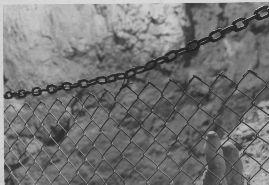
Photo 34. "Chicken wire" in Newdegate Cave. Where used to protect cave formations from vandalism, an alternative is perspex.
