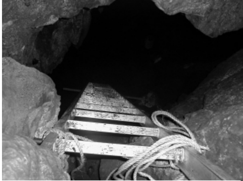
Figure 2: Aluminium ladder (with square rungs) leading down from new entrance gate in King George V Cave . Photo by Arthur Clarke.
