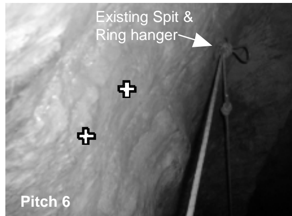
Pitch-heads (shown looking into the cave) in Midnight Hole showing the proposed sites (white crosses) for new P-hangers.
