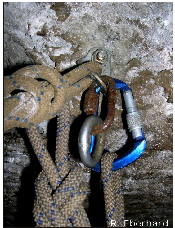
Plate 2. Fixed rigging in Ice Tube (December 2012). Note combination of stainless with other steel components.
