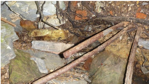
Eroded stone structure on the riverbank. Iron bars were used as reinforcing rods; pieces of brick were included.
