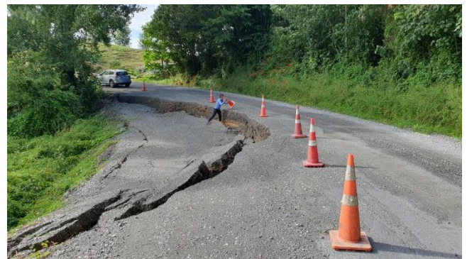
Roads damaged in all the rain (note the person in blue for scale). Photo: John Oxley
