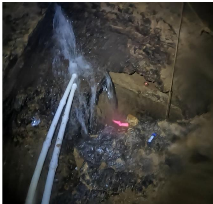
Water diversion across the pit using screwed-together pipe lengths. Photo: Stephen Fordyce
